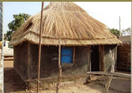
Finished hut roof with grass attached over the tarpaulins.
