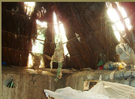
Damaged hut roof.
